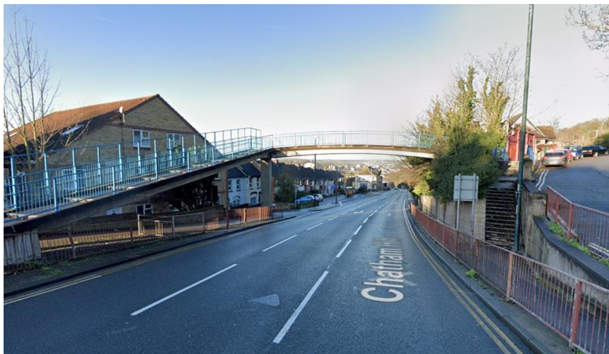
Figure A4.8: Chatham road, facing north-west towards Chatham town centre
