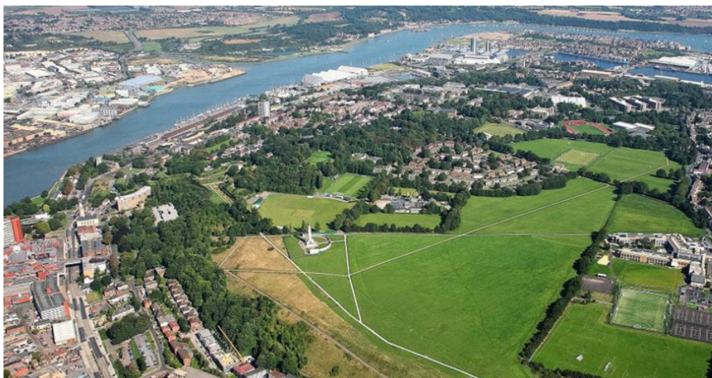
Figure A4.1: An aerial view of the Chatham Lines and the Dockyard 31
