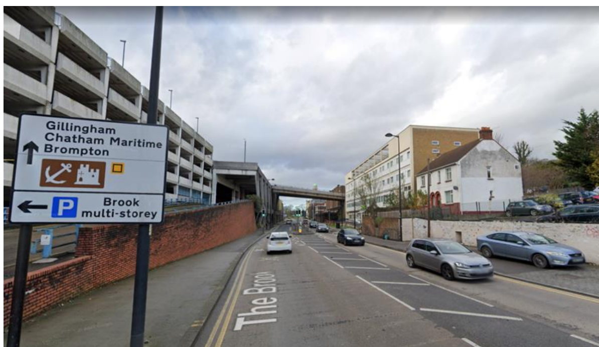
Figure A4.5: The Brook (A231), facing north west
